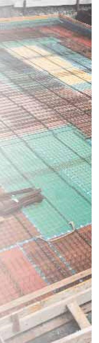
he bedding on Sylomer<sup>®</sup> can be full surface, on strips or on point bearings. The bearing design for the building depends on the specific natural frequency and the construction features. Connecting structures, such as ceilings or walls, can be of insitu concrete or can be prefabricated. When cast from in-situ concrete, the bedding surface is normally utilized as lost formwork. The reinforcement can be fitted directly on the mats. For
