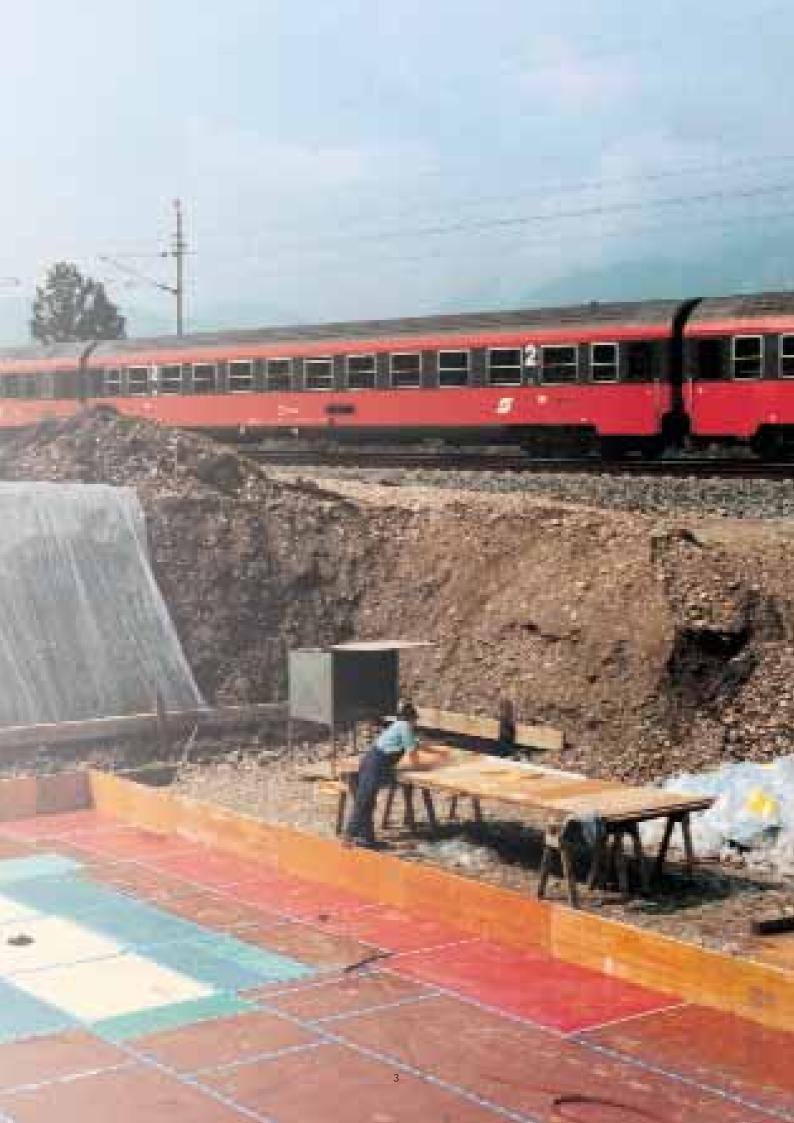
With Sylomer<sup>®</sup>, the designer has a technical material available for resilient bearing purposes, which suits a multitude of construction methods. The bedding can be provided over the full surface, in strips or at individual bearing points. The specific location at which the building must be resiliently separated is not predetermined for a bedding on Sylomer<sup>®</sup>. Separation is made wherever it is most favourable for the design.
