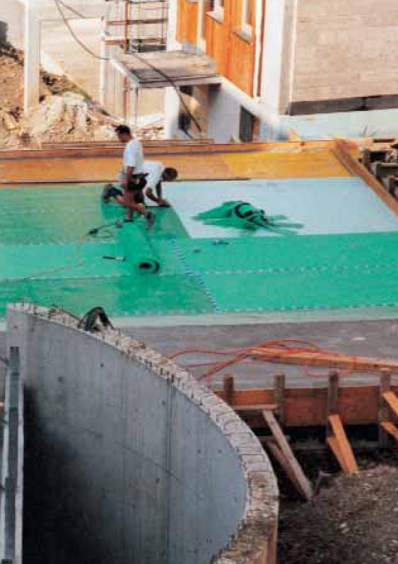
**S**ylomer<sup>®</sup> sheets and the bearings they form, are flexible and adapt to the contours of the foundation when loaded. The stiffness of the bearing depends on the load it supports and increases with this accordingly.
