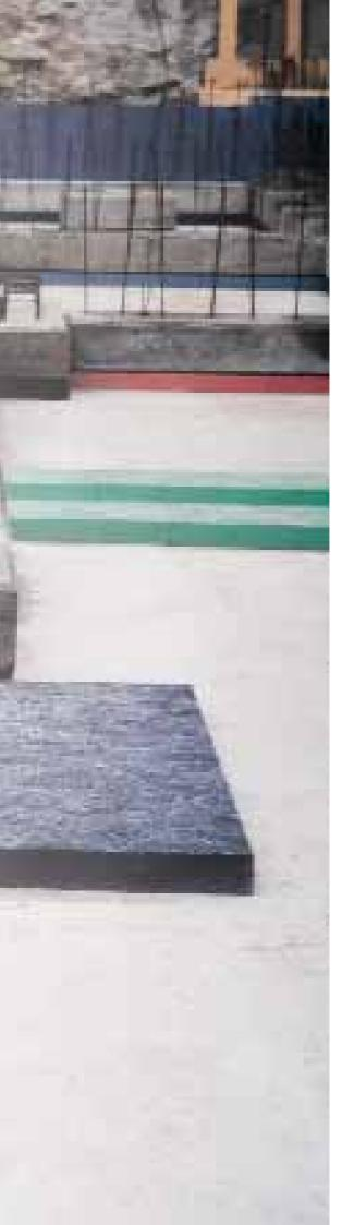
Sylomer<sup>®</sup> bedding is supplied to site in sheets or cut to size as individual bearings. Cutting on site is possible with standard tools.
