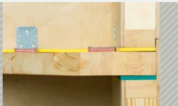
Elastic mounting of walls and ceilings
